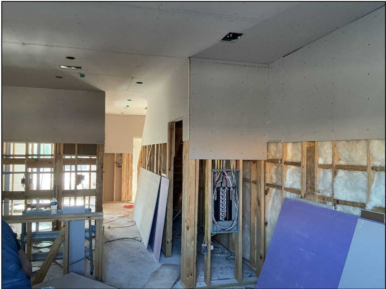
Unit Interior Drywall Installation
